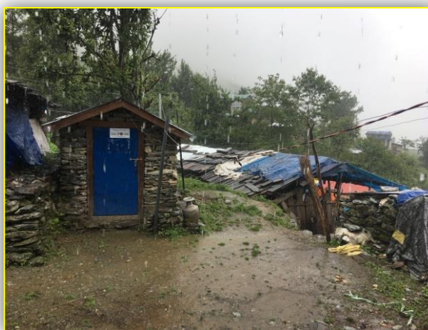
Repair of HHC built Toilet in Tipling Village
