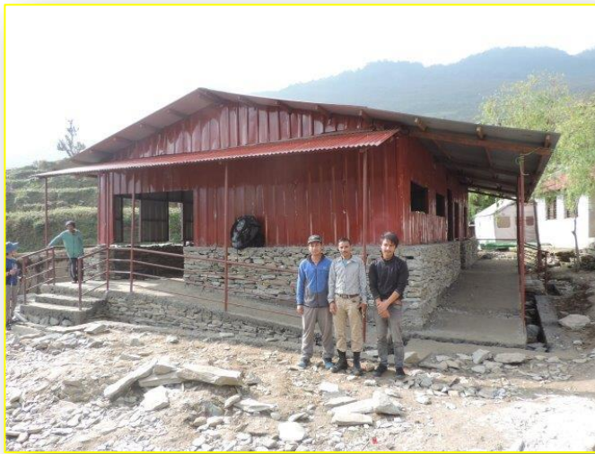
Lapa Village Health Post Reconstruction (one of eight)
