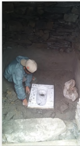
Toilet recipient setting the ceramic pan
