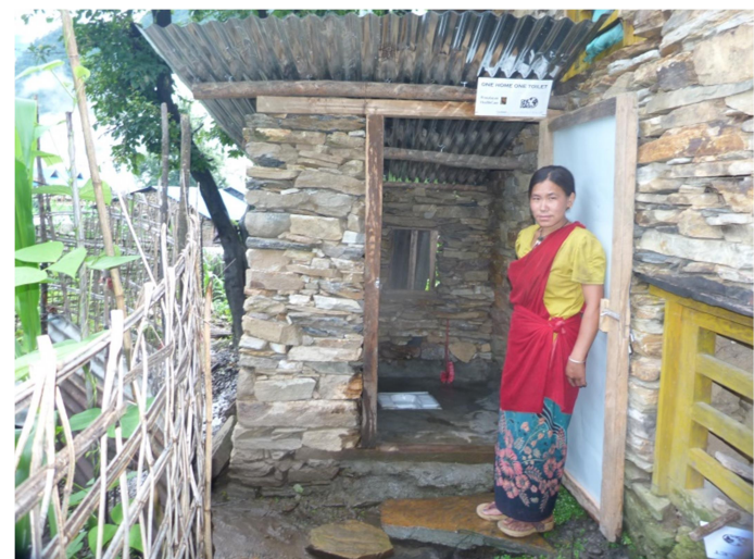
HHC completed 100 toilets in July 2020. A proud new owner in front of her toilet in her home in Sertung village
