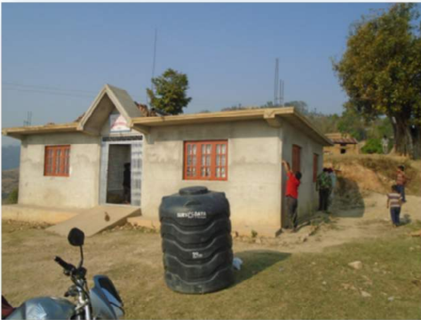
Bhumisthan health post before repair
