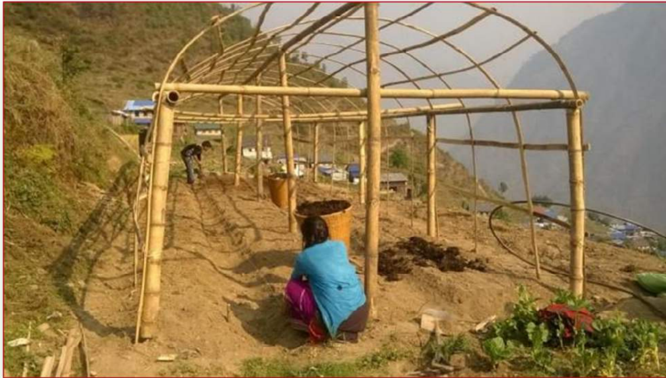
Building a greenhouse at HHC experimental farm using local materials
