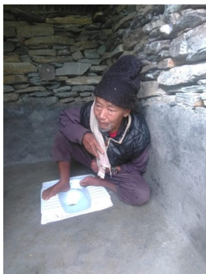
Paralyzed Sertung man, receiving a permanent toilet, appreciating his new life-changing facility as installation was completed.
