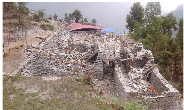
Figure 1 two hostel building after earthquake
